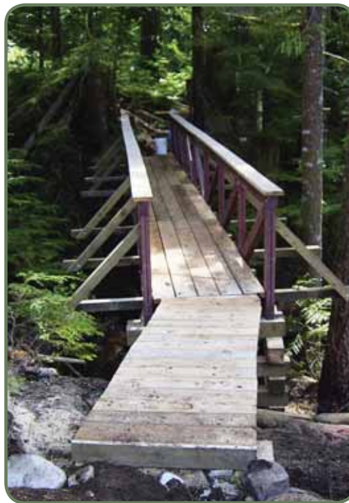
Photo George's Crossing Bridge Courtesy of Todd Pope
